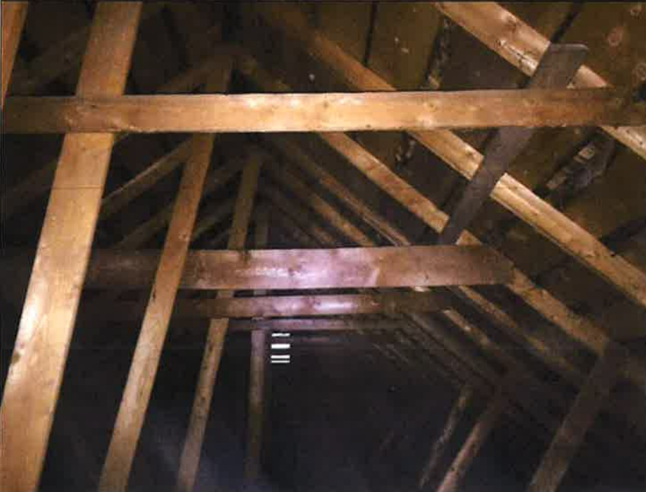
Photo 6: Roof rafters looking north from access hatch
