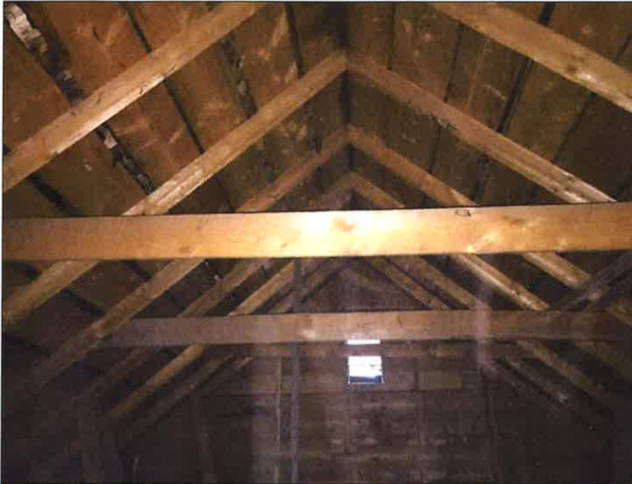
Photo 5: Roof rafters looking south from access hatch
