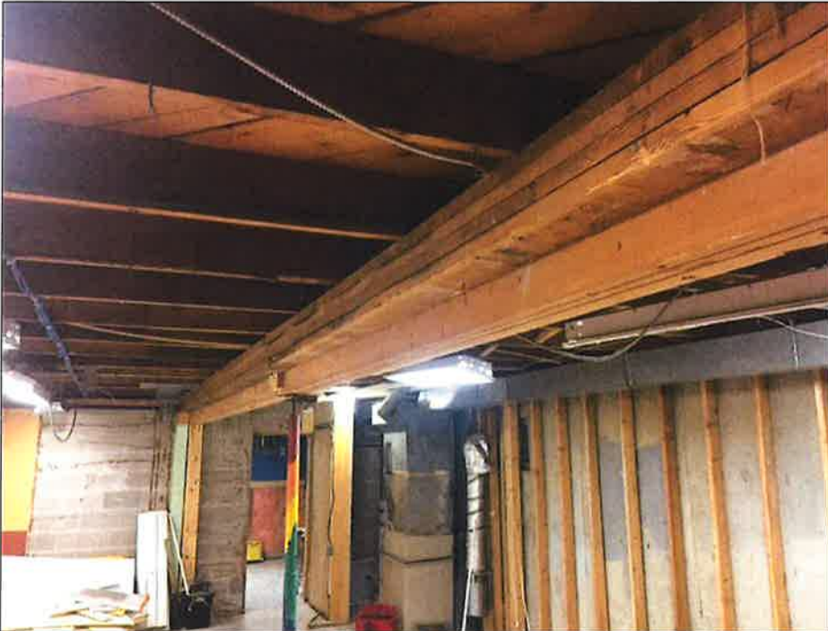
Photo 7: Intermediate support beam – Note side laminated sister beam
