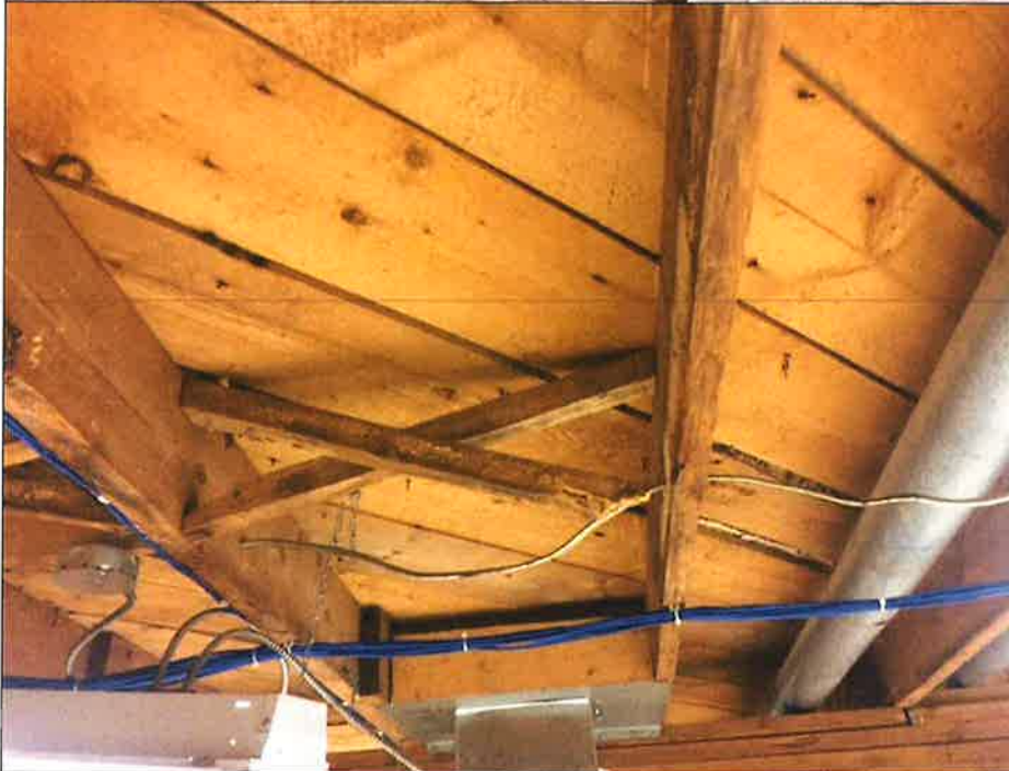
Photo 10: Typical floor joists and decking
