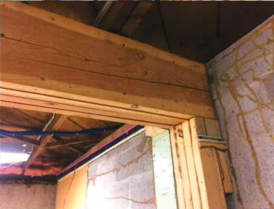
Photo 8: Typical intermediate support beam bearing on 4-ply post (top connection)
