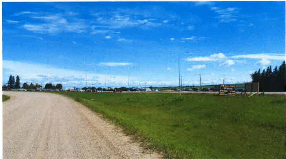
Proposed Location 1, Photo 1 - North facing view of Road Plan 8822959 from Range Road 23
